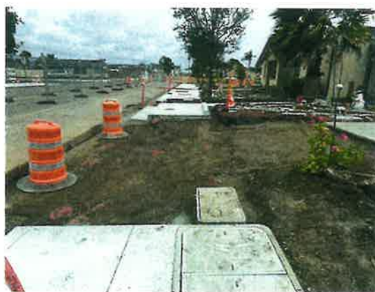
Photo of recent project work near State Route 183 in Castroville.
